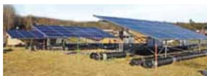
Anar Solar's racking system via clamps. The racking supports 20 panels in landscape orientation at between three and nine feet (0.9-2.7 meters) of elevation.
